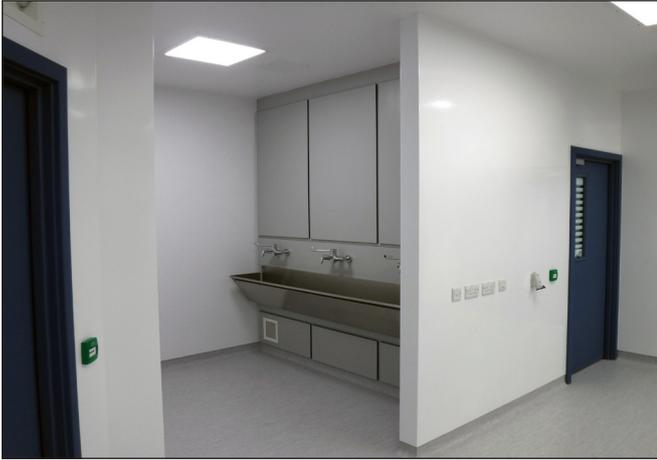
**8.46** Where the scrub is a trough on the wall or in an open bay within the operating theatre, it should have low-level extract under it.
