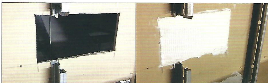
Here (left) a contractor has made an aperture for the subsequent installation of ventilation ducting, but, as shown (right), the installer has subsequently selected a different location for the ducting. There is a clear need to regularly inspect all compartmentation to ensure that protection remains in place and appropriate.
